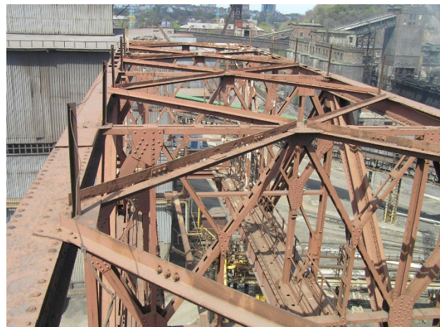
Fig. 4. Upper bracing trusses of the crane's span structure
